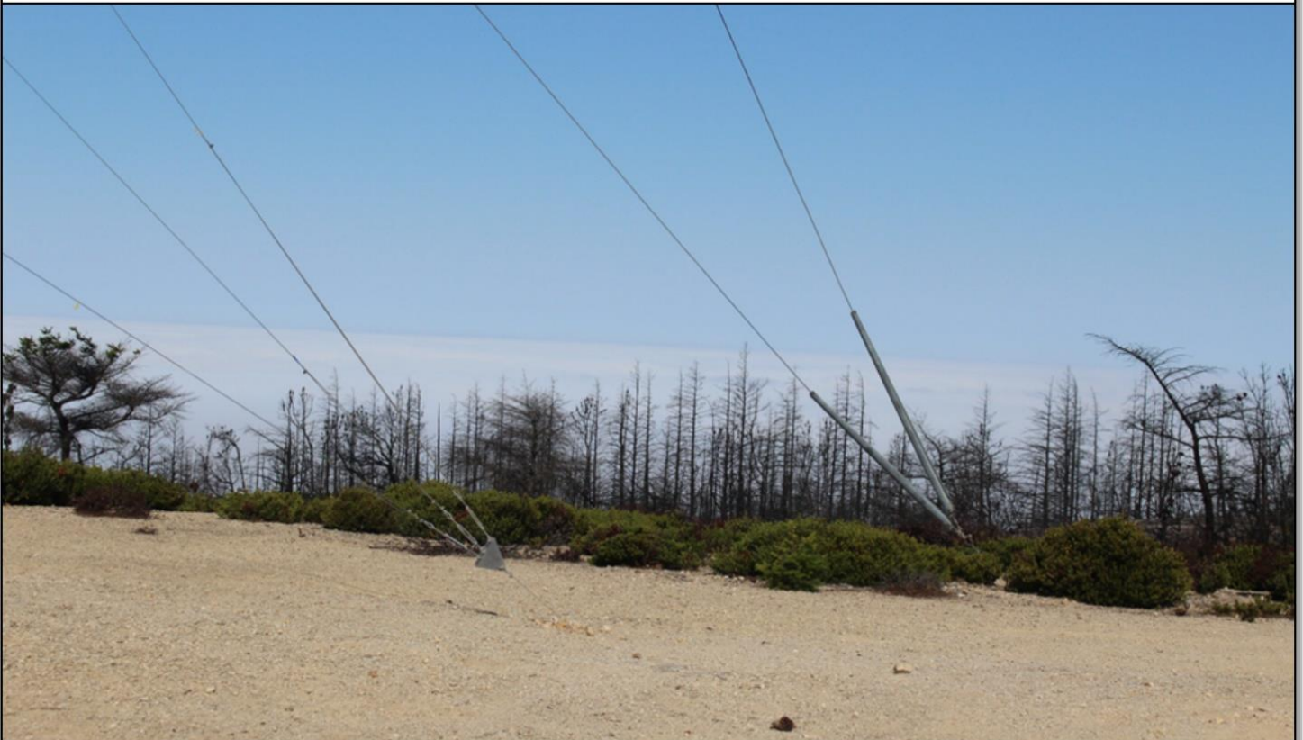
View from Project Site looking West
