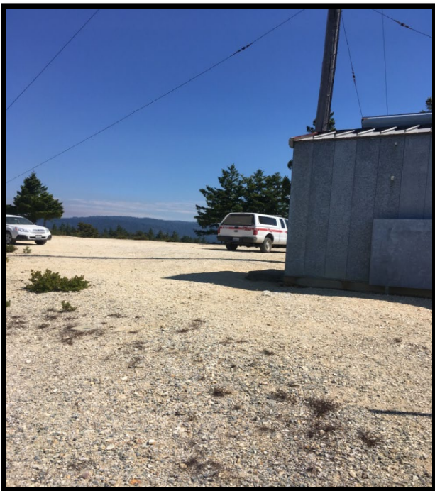
Photo 7: Existing facilities at Chalk Mountain.
