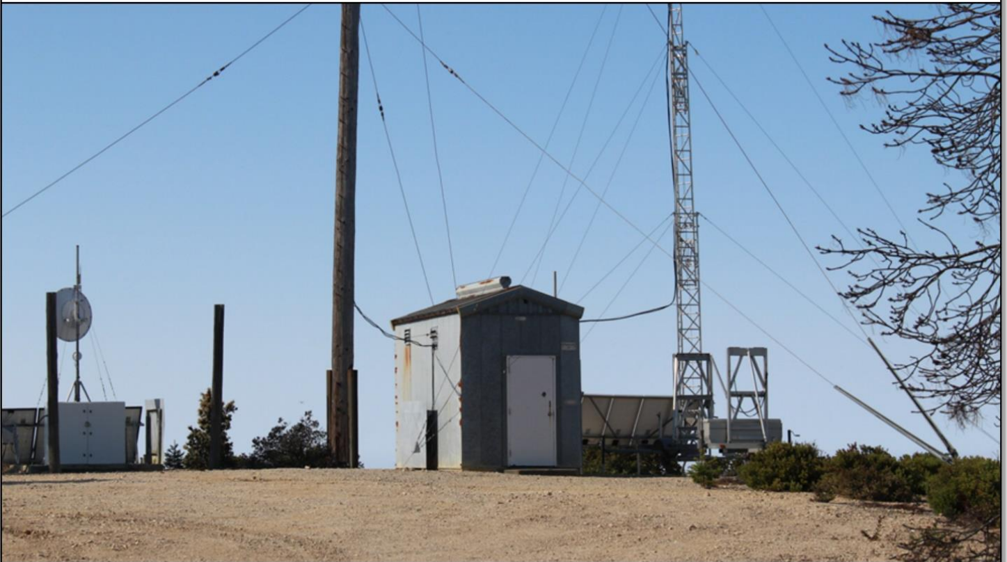
View of Existing Facilities at Project Site looking South
