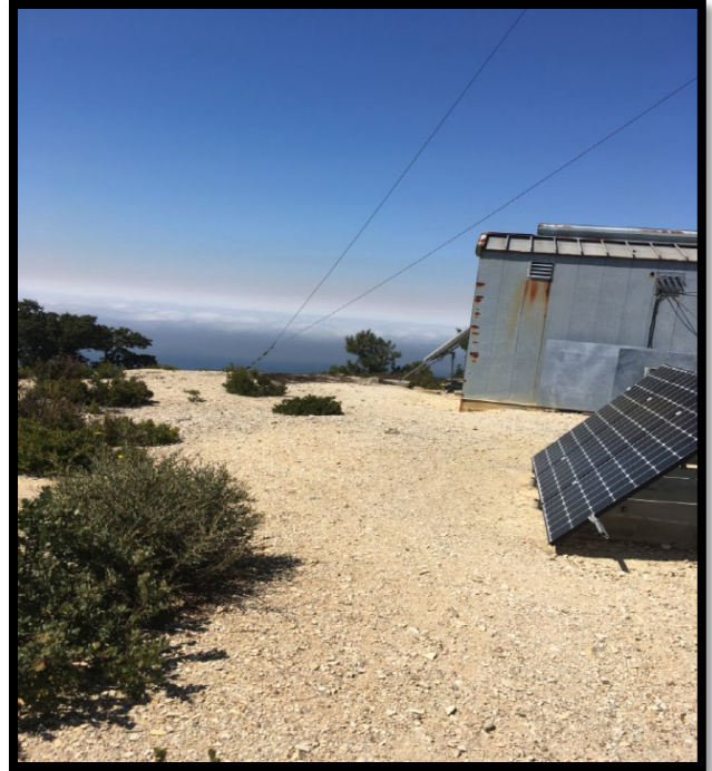
Photo 6: Existing facilities at Chalk Mountain.
