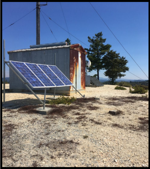
Photo 5: Existing facilities at Chalk Mountain.
