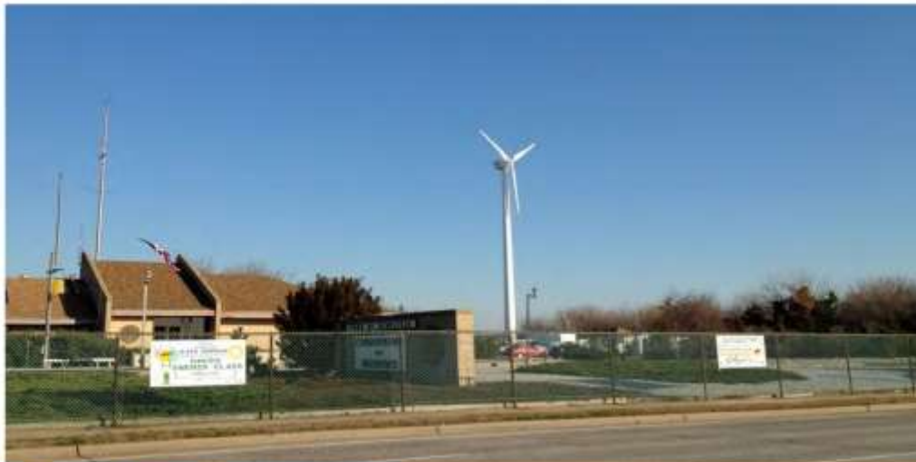
Northwind 100, 100-kW wind turbine; Hempstead, New York. Photo by Town of Hempstead, NREL 28963
