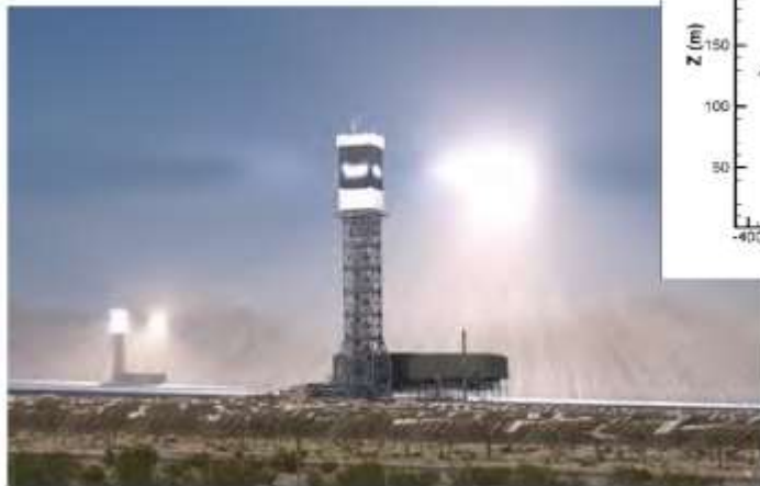
Photo and model of high-flux regions causing solar glare and avian hazards at Ivanpah Solar Electric Generating System
