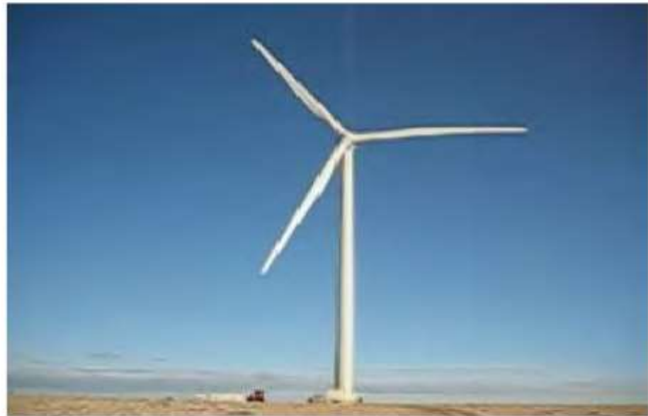
93-m diameter RSA and 2.5 MW
