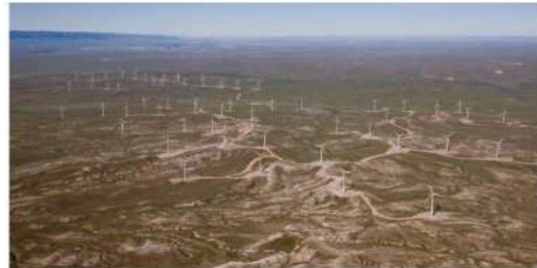
An aerial view of Duke's Top of the World wind farm, located in Casper, Wyo. Photo courtesy of Duke Energy Renewables
