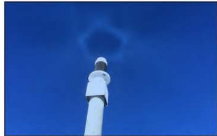
Figure 1 – The halo created by the reflected light of 3,000 heliostats which caused the bird mortalities.
