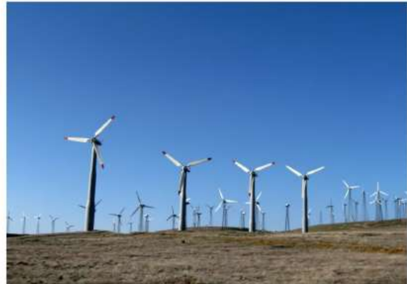
705-MW project in Tehachapi Pass Wind Resource Area, California.
