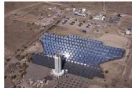
National Solar Thermal Test Facility (NSTTF)
