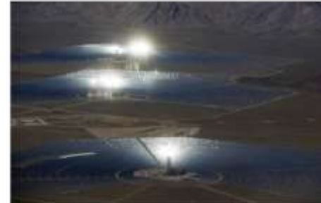
Ivanpah Solar Electric Generating System
