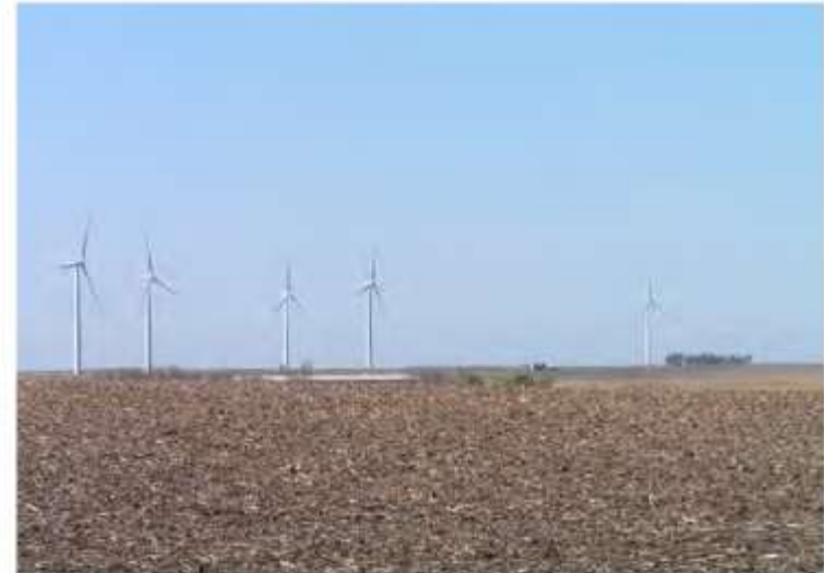
Junction Hill Top Wind Farm, Iowa. Five GE 1.6-megawatt (MW) turbines. Photo by Tom Wind, NREL 26494
